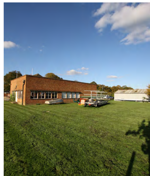
QBC Gym/Tank Room 2017
